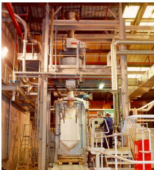
The Webster Griffin control panel and wiring are intrinsically safe and owing to the low melting temperature of the powder, overheating of any component or motor is monitored automatically, the motors are also explosion proof.
